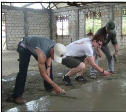
Stephen helping smooth cement
